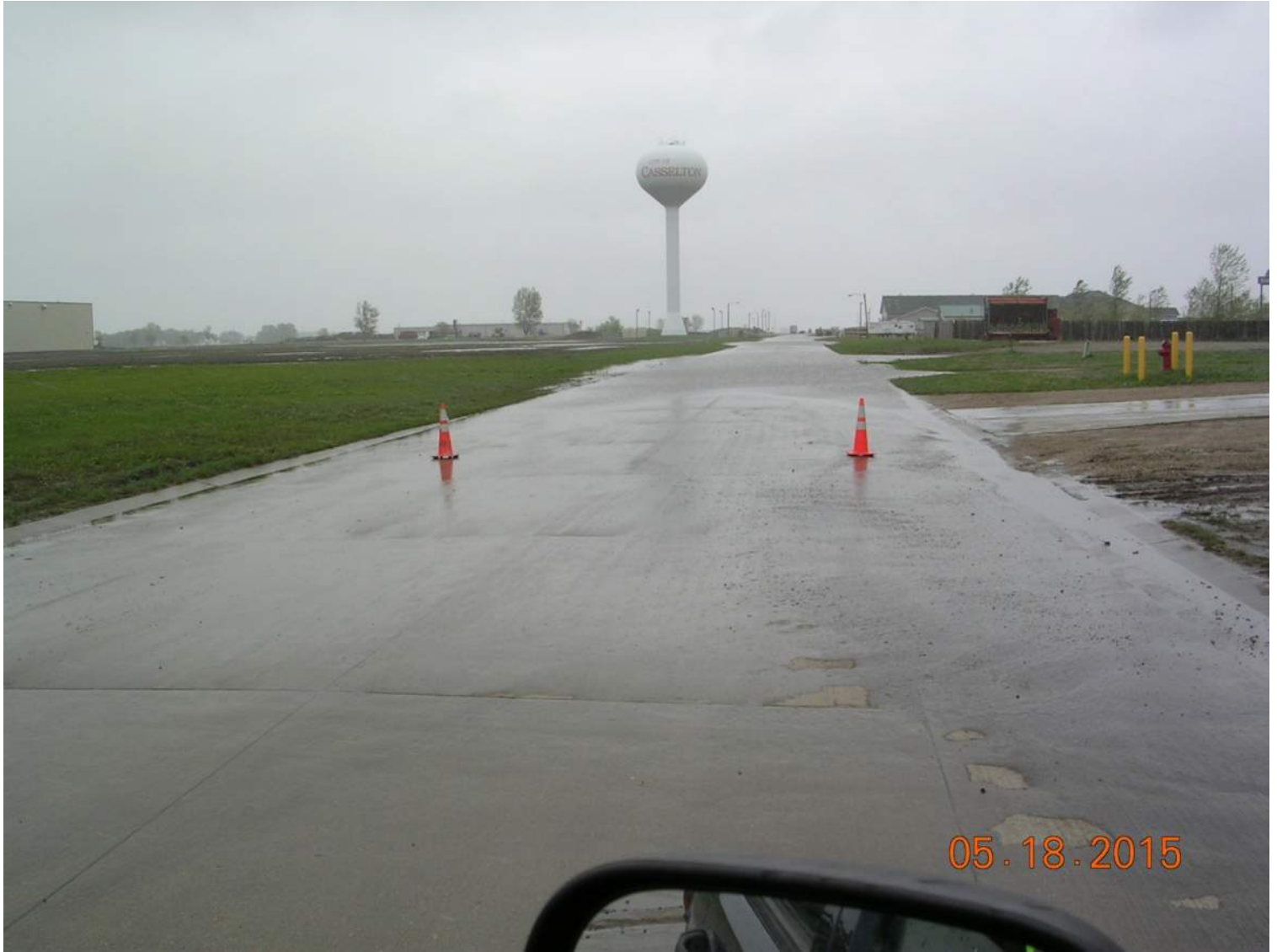
Industrial Boulevard during rain event (looking east)
